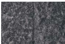
F058 Blocked Slate
